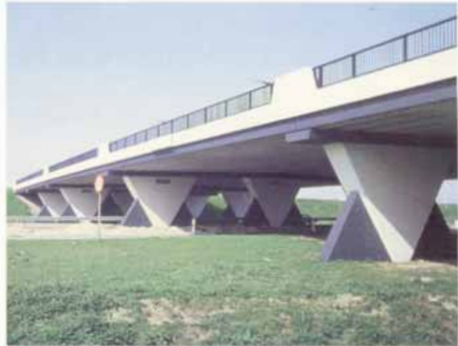
Figs. 1. Bridges in the dutch countryside – an old (a) and a new precast concrete bridge with white coloured concrete (b)
