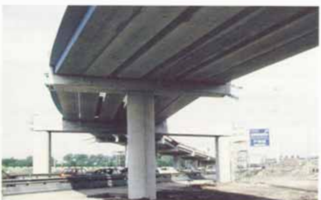
Figs. 2. Cast-in-situ bridge, extended formwork a hinder for the traffic (a) an a precast bridge a minimum of hinder for the traffic (b)
